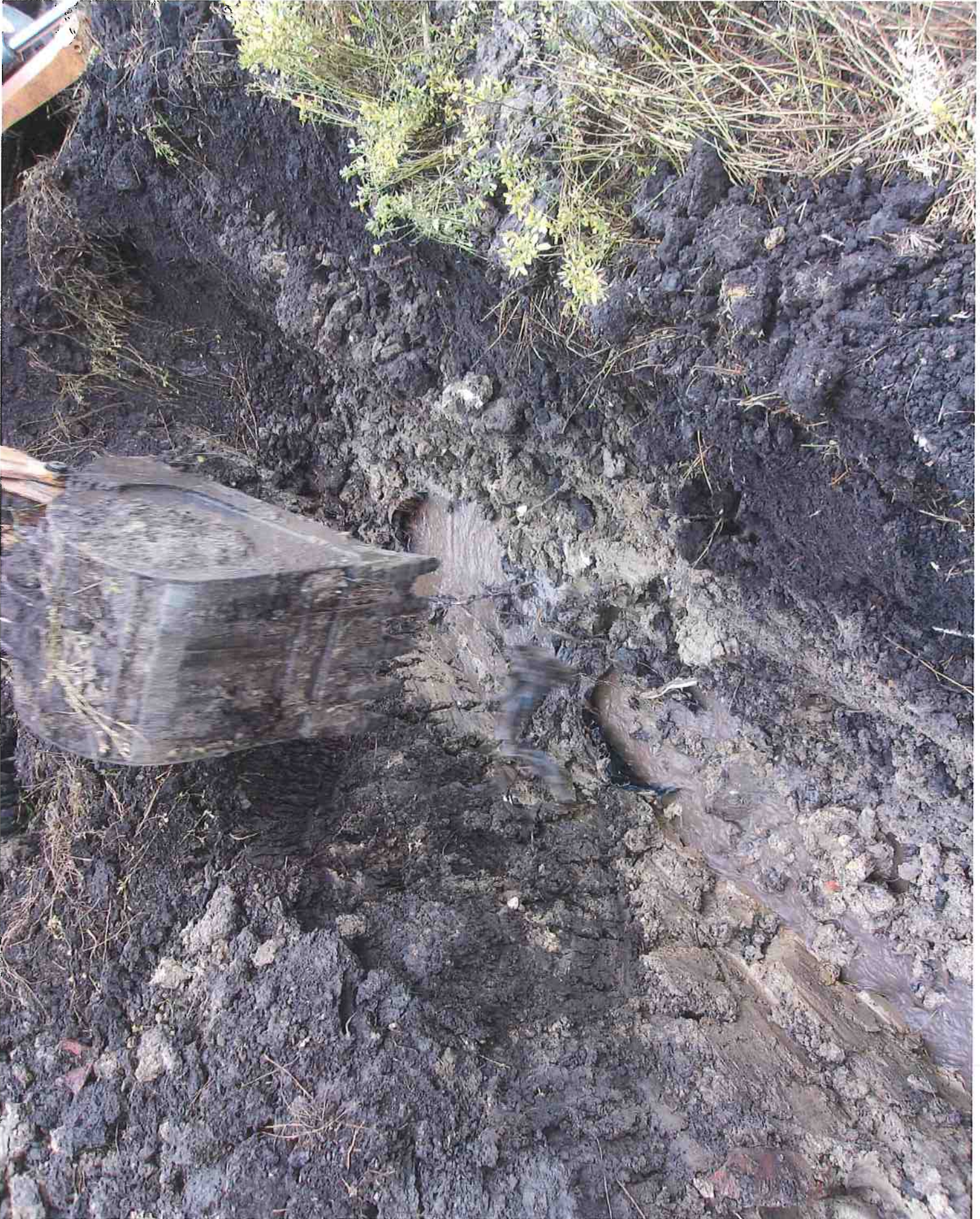
REMOVING 63' OF 12" PE TILE WITH ROOTS THRU TILE WALL
