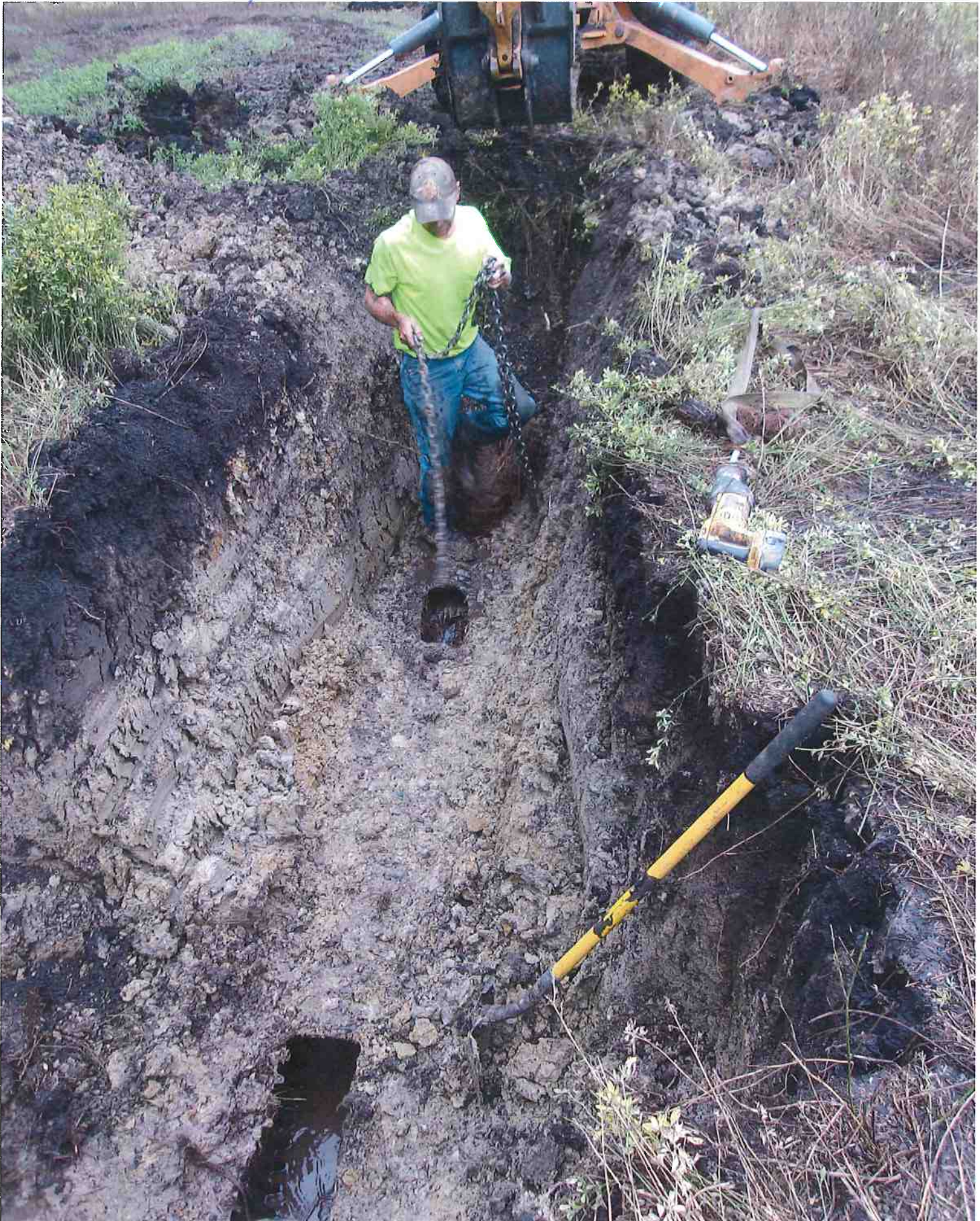
Hooking up LOG CHAIN TO ROOTS IN TREE
